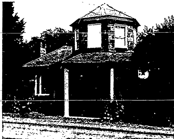
Addison tollhouse on the National Road (now U.S. 40) in Somerset County.
