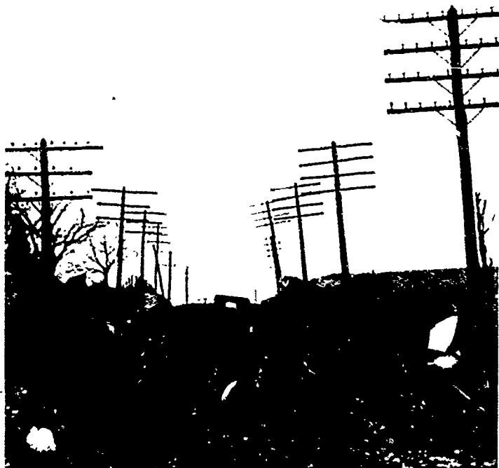
This road in South Fayette Township, Allegheny County, was a sea of mud in early April, 1916.
